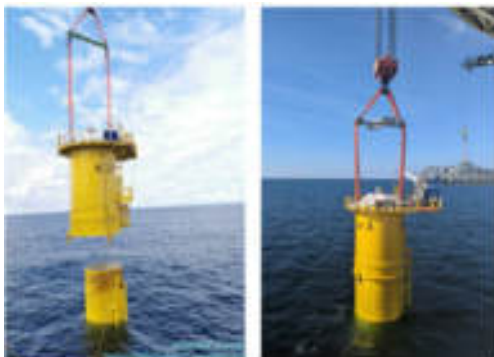
Figure 1: Monopile foundation installed at KASKASI-II wind farm, © RWE AG
